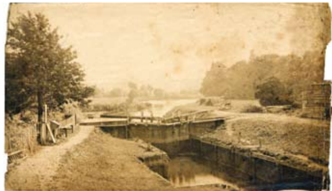
This early photograph of a turf-sided lock shows how they appeared by the mid-nineteenth century, after they were widened to take Newbury barges. Today only Garston Lock, of which this may be a picture, gives any idea of what it was like to use such a lock.
