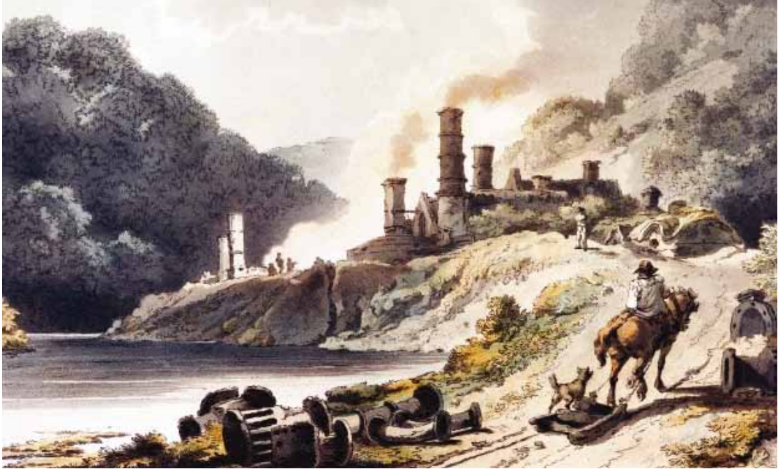
▲ The Madeley Wood (or Bedlam) Ironworks was built in the late 1750s on the north bank of the river Severn a short distance from where the Iron Bridge was constructed some 20 years later. It was one of five groups of coke-fired blast furnaces built in the Shropshire Coalfield within less than five years, which marked a real revolution in the pattern of iron making in England. This view depicts the furnaces from downstream and shows in the foreground a sled, apparently being used to transport coal. Probate inventories confirm that the use of sleds was not uncommon in this part of Shropshire in the early eighteenth century.
